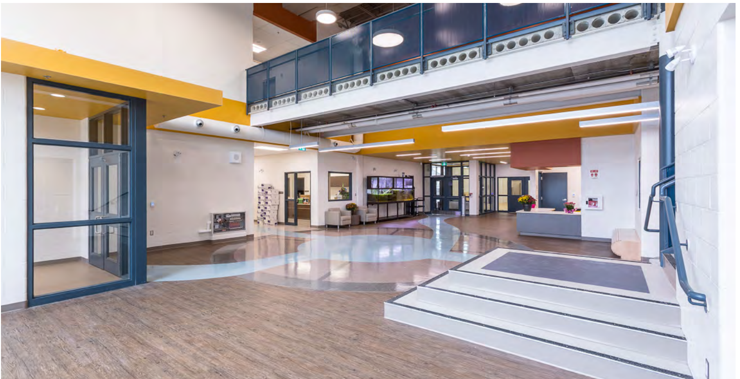
▲ Main Entrance and Entry Commons with second storey catwalk. Structural systems and hollowcore slabs are left exposed as a teaching opportunity.
