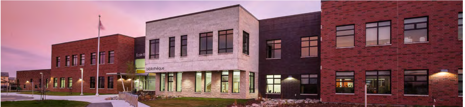
▲ Front elevation with the Learning Commons / Library front and centre.
