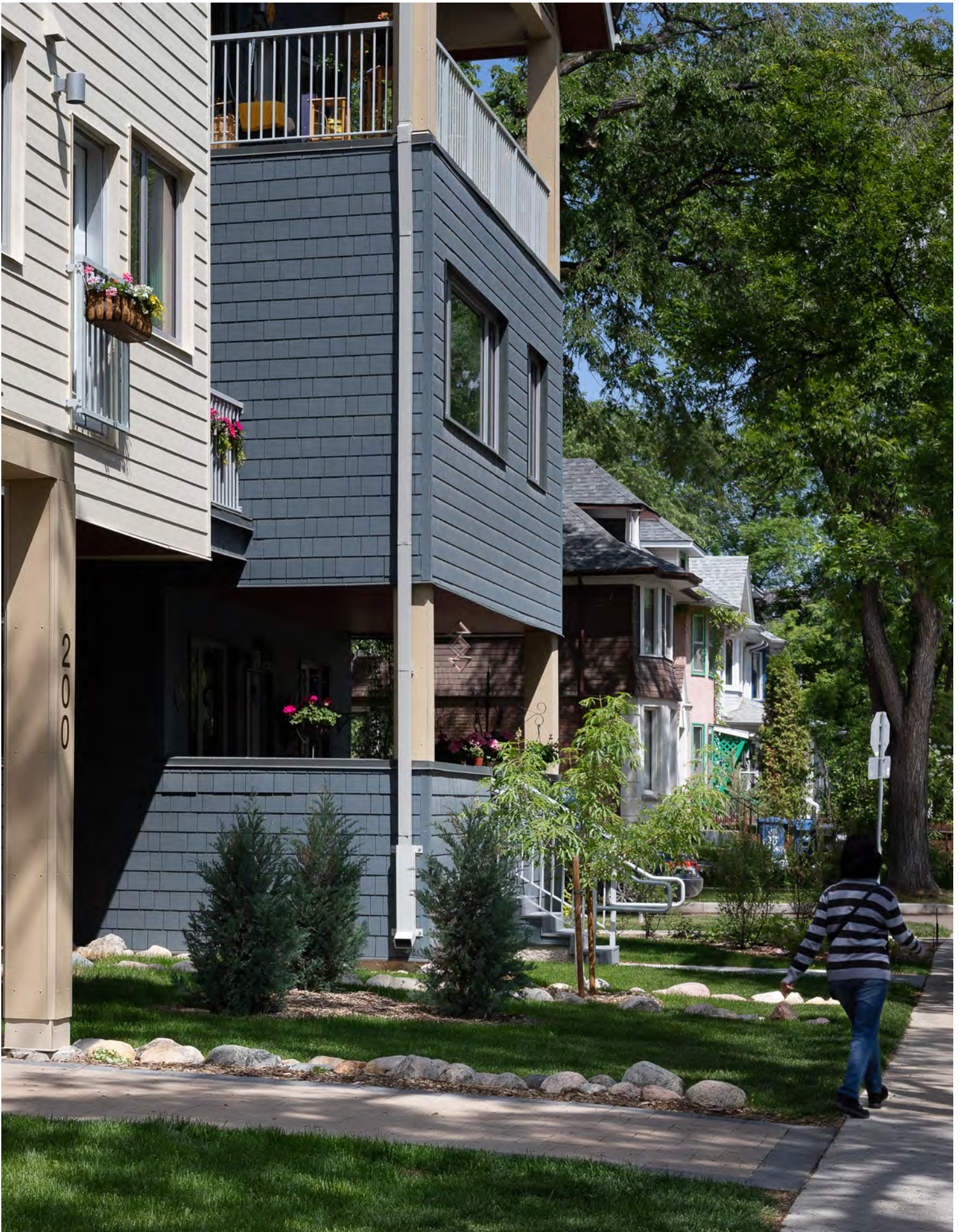
▲ View of the Arlington Street elevation, looking north towards existing homes that represent the residential character of the neighbourhood.
