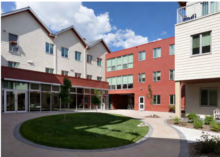
▲ View of the covered Arlington St. entrance and Commons from the courtyard.
