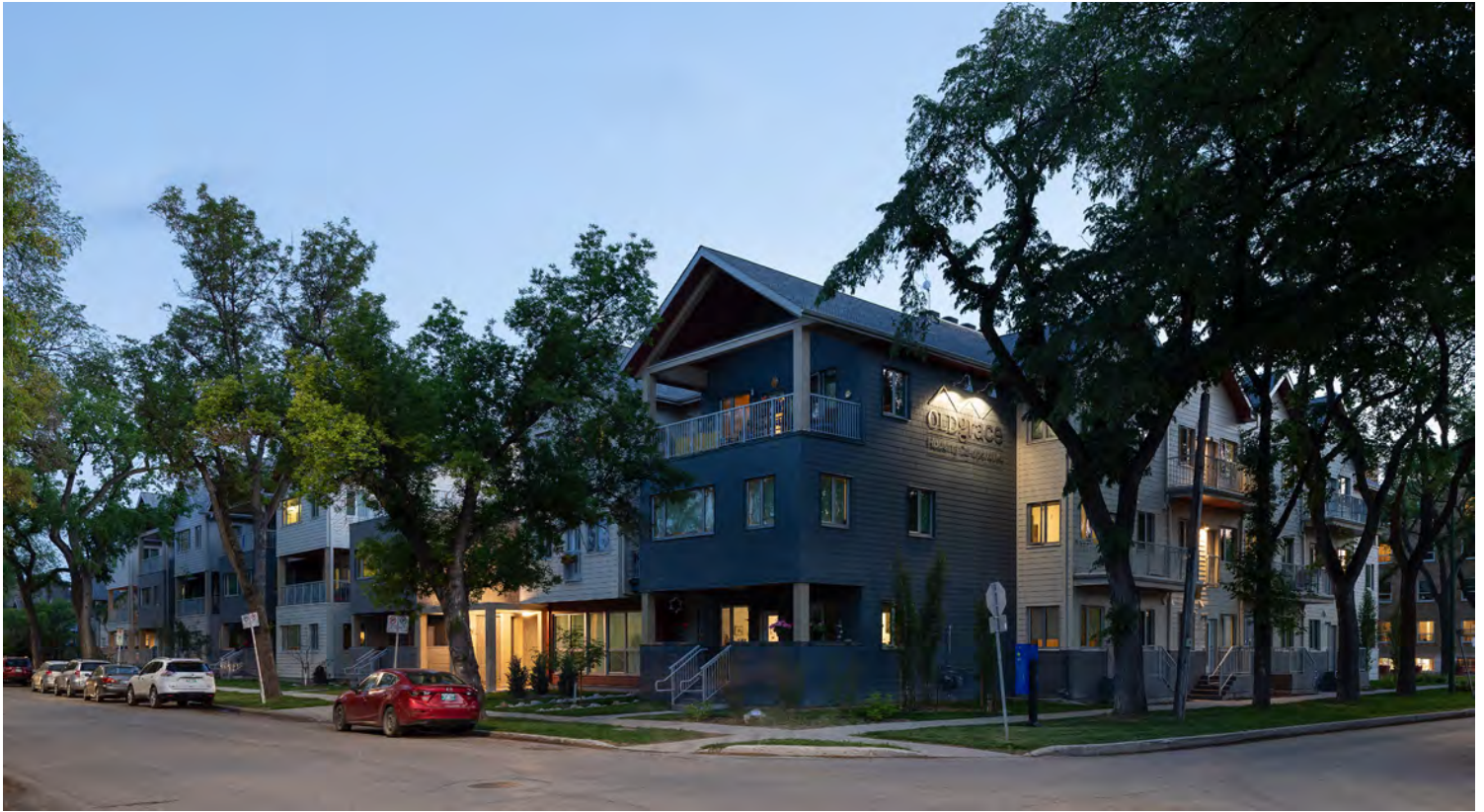
▲ Evening view from the corner of Arlington Street and Preston Avenue. A careful lighting strategy accents the entrance and building signage, but minimizes light pollution.
