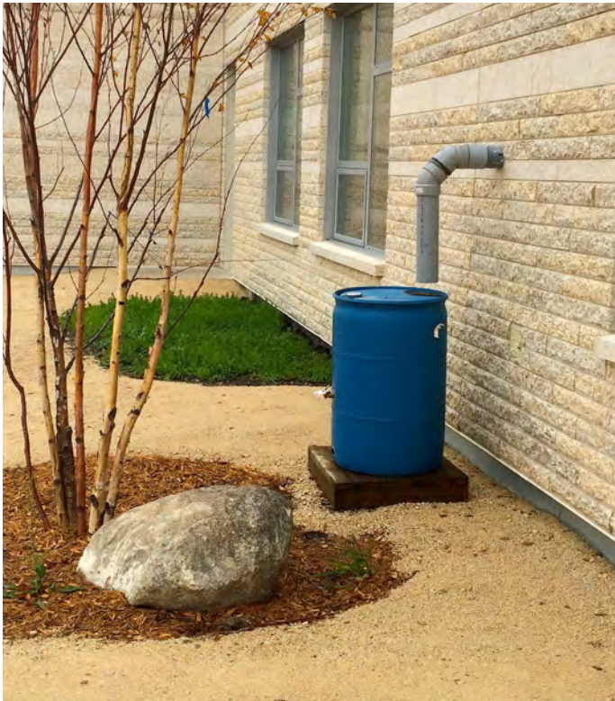
▲ Harvesting rain-water reduces the water use of the O.L.E. and landscaping even further.
