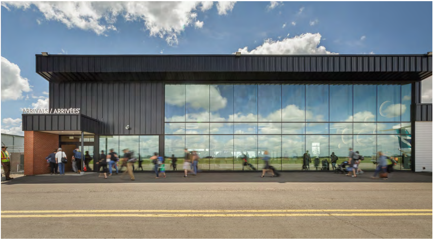
▲ Arrivals entrance and large arrivals hall glazing as seen from the runway.
